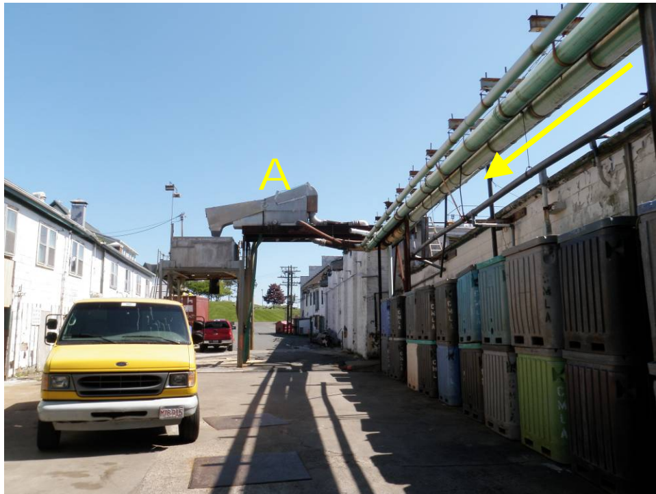
Figure 11. When a boat offloads at this port the herring move in the pipes, some 20 feet off the ground (yellow arrow), into the dewatering box (A) and then into a truck (not pictured).
